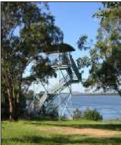
The observation tower at Hooka Point looking over Koong Burry Bay
