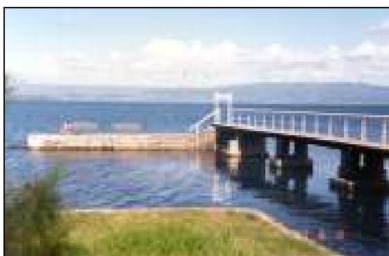
Dixs Wharf after initial restoration
